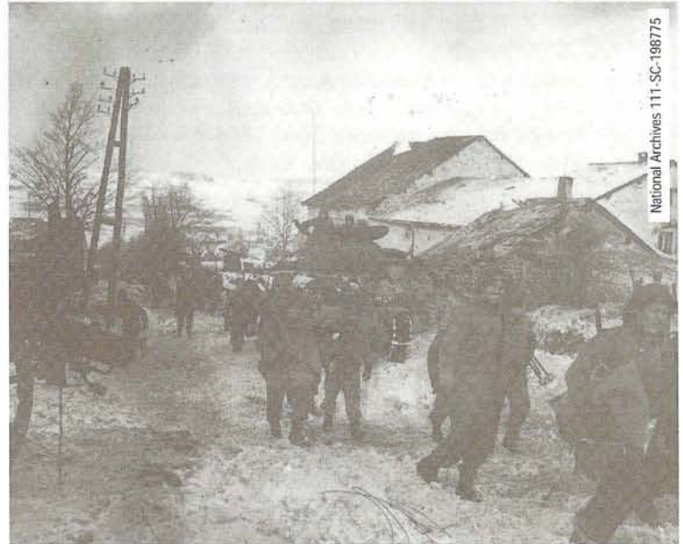
The off-recurring scene of Americans moving through a Belgian town to attack Germans dug into positions beyond the town. Here, the 87th Infantry Division moves through Biheine.
