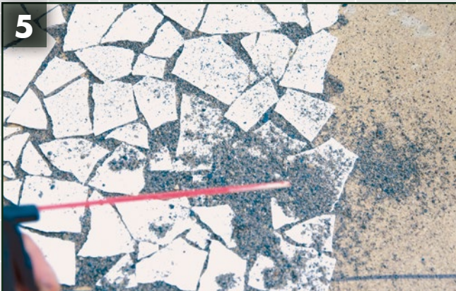
Step 4) Sprinkle play sand over the whole area. Be sure it gets in all the crevasses.
