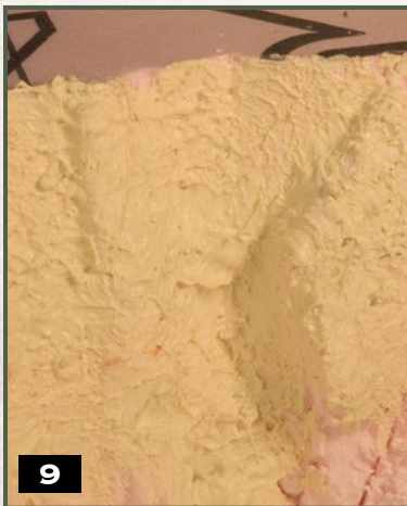
9 Step 9.) When the spackle dries, put on the leather gloves and rub off all those little peaks. Continue until you achieve the look you want.
