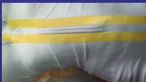
Zip area masked off prior to applying putty
