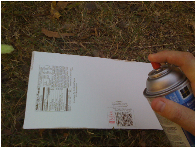
Spray a single, even coat of epoxy on the cardboard surface.
