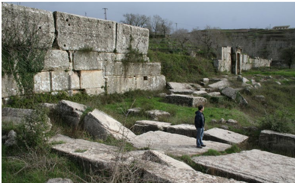
The cyclopean wall blocks that have collapsed inward to the east of the north entrance, with the eastern entrance in the background
