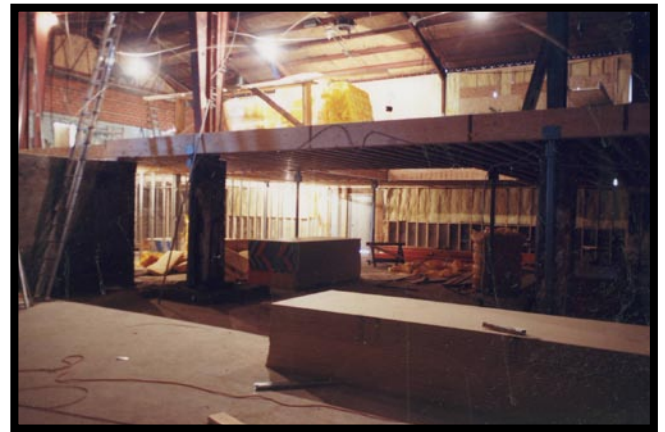
Putting the floors
