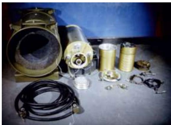
Above: Case (left) and internal components of the W45.
