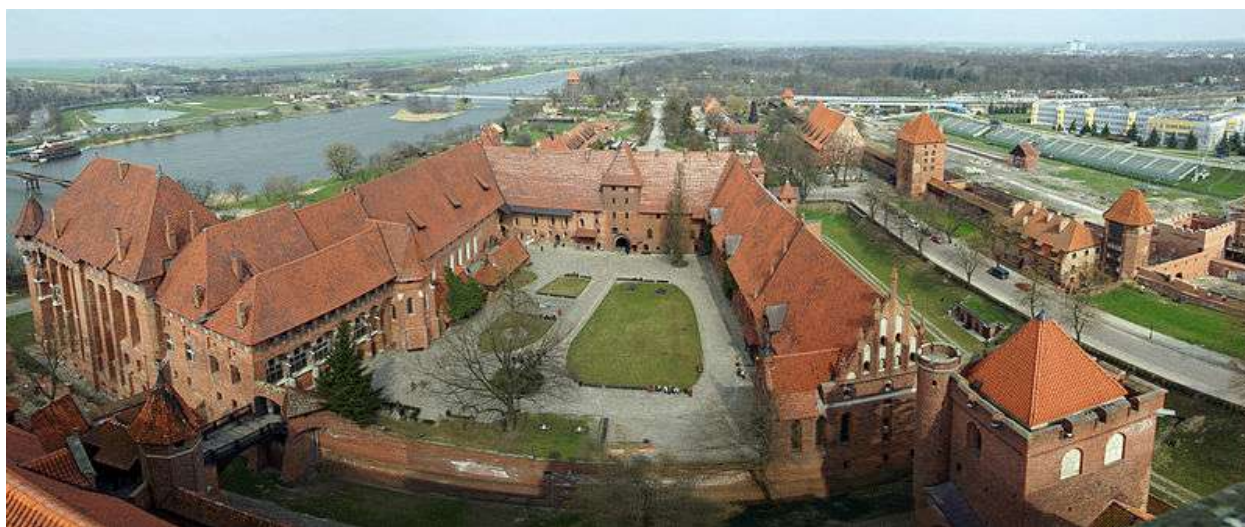
Above: A view north from the High Tower over the Upper Castle, looking down on the Middle Castle and the Lower Castle beyond, as it looked in early 1996. On the right, from the foreground: the District Governor's House, the Carved Gate, and the armory. The Nogat River is on the left of the picture; Malbork city is on the right.
