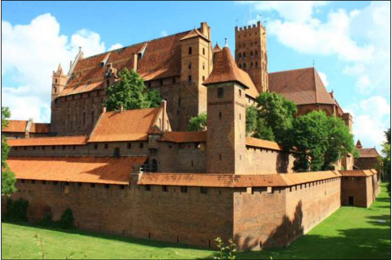
Above: A view of the southeast corner of the High Castle from beyond the outer wall, atop which the covered hoardings are clearly visible.
