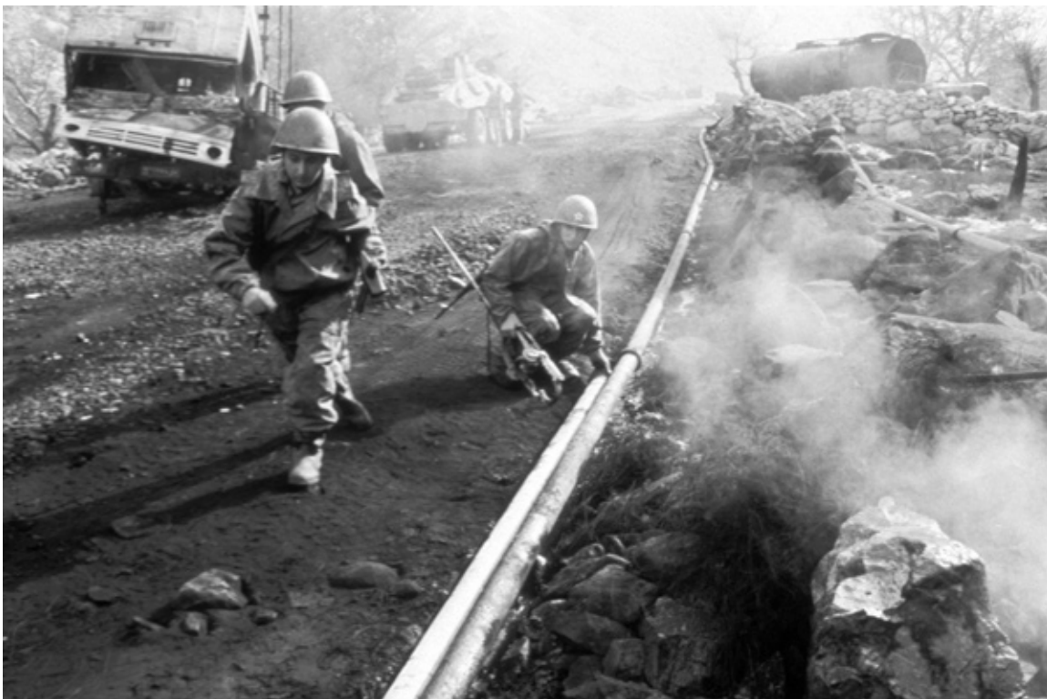
Pipeline troops inspect 4 th Czechoslovak Army's main fuel pipeline following a NATO air strike, Northern Bohemia, July 1997.
