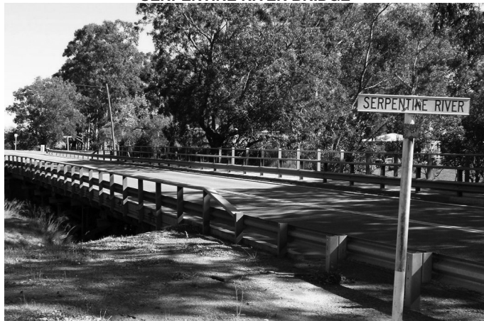
SERPENTINE RIVER BRIDGE
