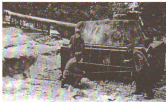
A descriptive photo of the boxed Panther turret, aka "Pantherturn" being emplaced on the battlefield by German engineers.
