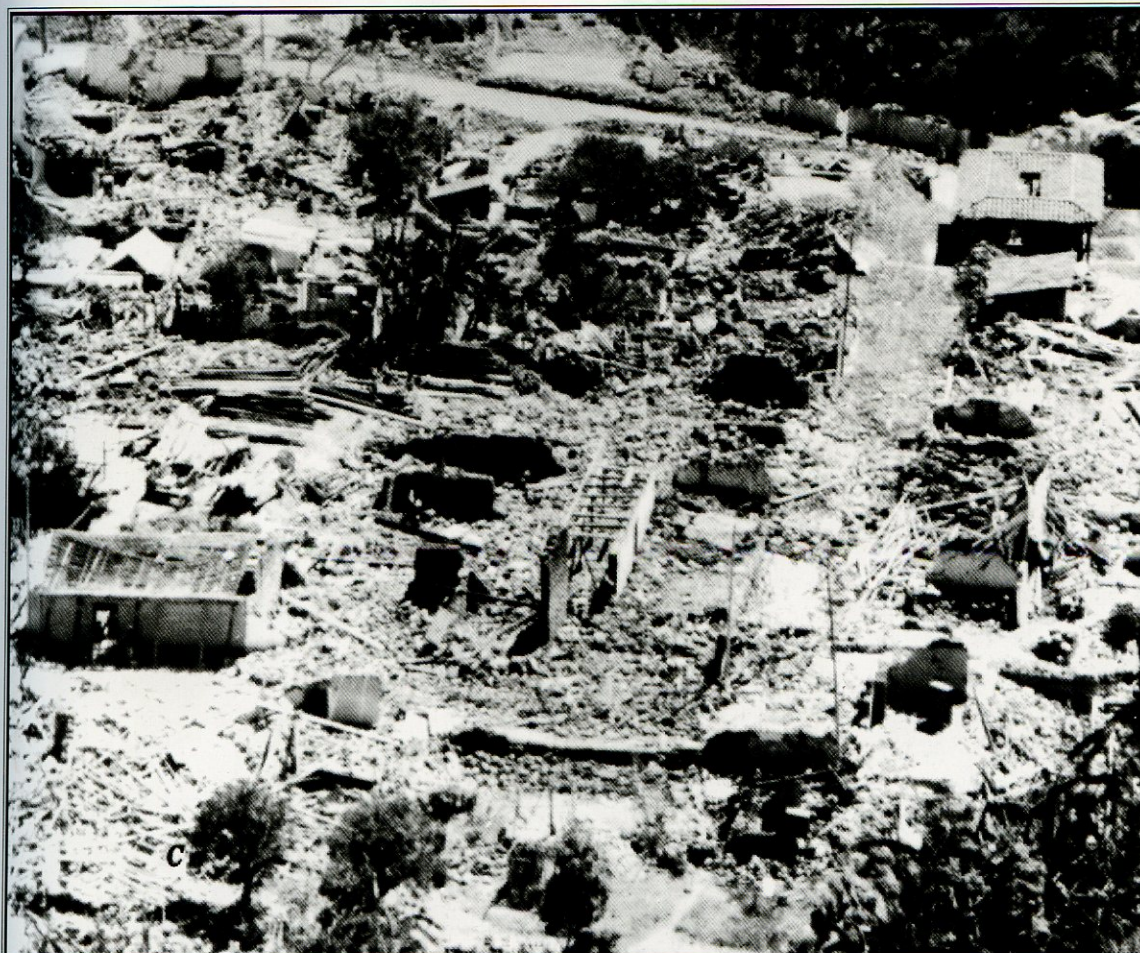
(Left) Devastated outer habs, Bal Prime.
