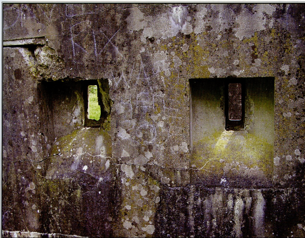
(Left) Abandoned pill-box defenses at Balopolis. Note the rockcrete/ply construction.
